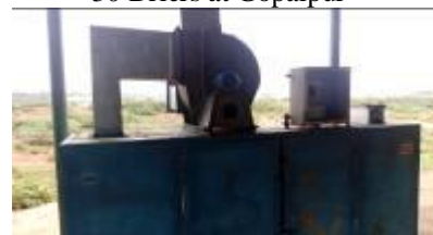
Drier with electrical equipments stolen
