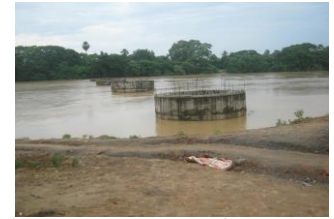
HL bridge at 3 rd km of Barachana-Balichandrapur Road
