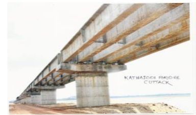
Kathajodi Bridge, Cuttack
